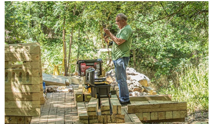
Sherwood Bishop working on the Matilda Bridge in San Marcos, Texas.
