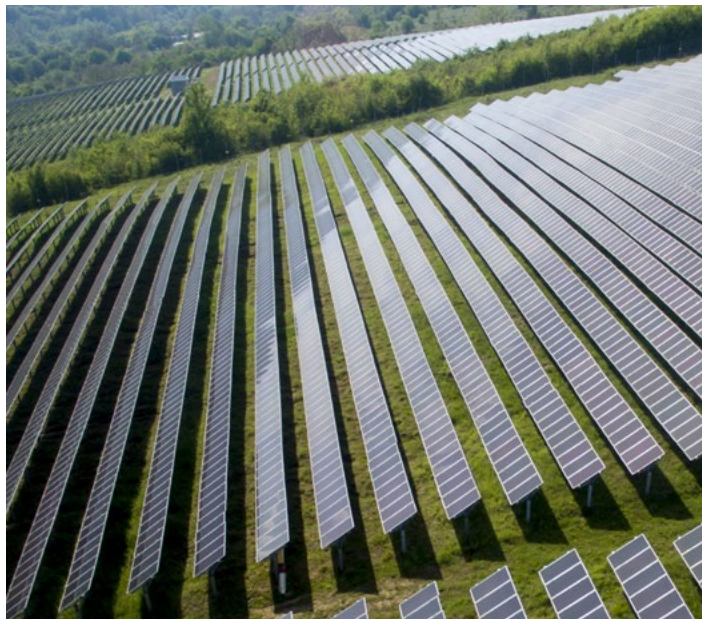
Aerial view of a Cox solar farm.
