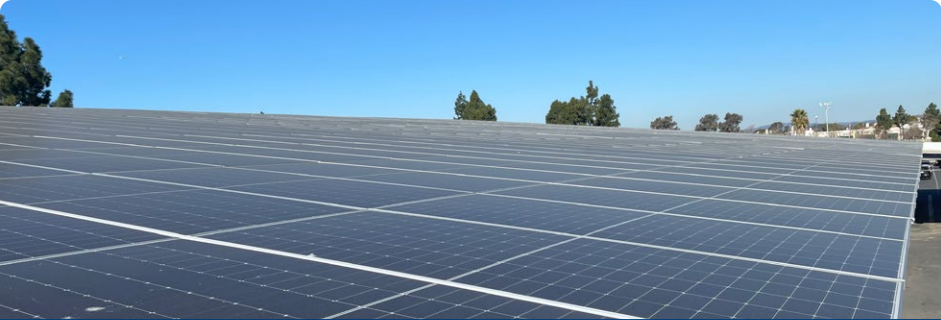
Solar canopies at Manheim San Francisco, California generates renewable energy to power vehicle inspections and support EV charging infrastructure.
