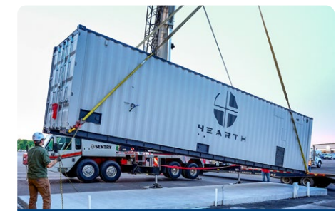
4Earth's smart, modular water reclamation technology being installed at Manheim Nashville.
